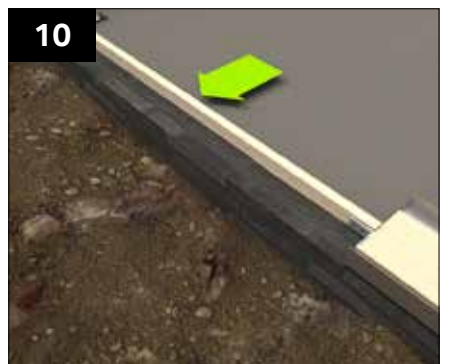
10 These trays can then be temporarily joined together using the provided set out battens and the tray steels as a datum, this step is optional primarily to assist with accurate tray positioning. Refer to you base plan for set out sizes
