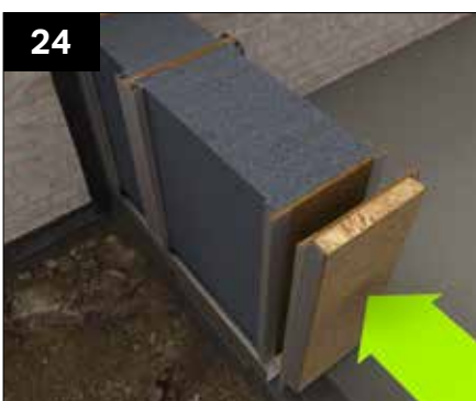
When an opening in the wall is reached, an aperture panel is used to terminate and allow for secure window fixing. Locate the relevant aperture panel and position this against a walling panel, as shown on the location plan.
