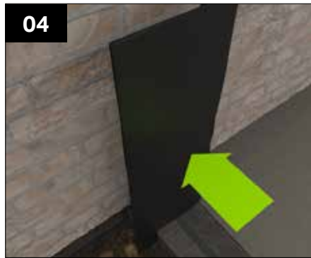
04 Insert the DPC into the channel created, this will require folding into an 'L' shape, the DPC may require cutting to seat correctly. Use packers to keep the DPC in place. Once the walling panels are fitted this will then be folded again to form a 'Z' shape. If required repeat this and the previous two steps on other junctions with the existing structure.
