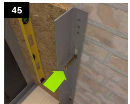
Ensuring the host wall tray is plumb and level, using the hinged element of the host wall tray secure into the host wall. When fixing into the host wall, ensure that the fixings are positioned to the bottom of the slotted hole as shown to allow the tray to lower once the skids are removed
