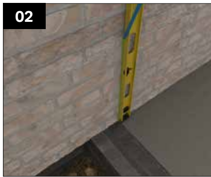
02 Where the walling panels abut the host wall a vertical DPC (NOT SUPPLIED) is required. To mark the position, strike a vertical line at the inside face of the outercourse of the foundation brickwork (or 100mm in from external base).
