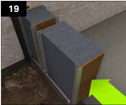
Position the following panel against the previous panel.
