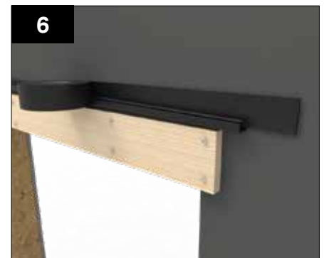
6 Using tape provided seal along the joint at the top between the soaker trim and the membrane.
