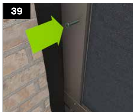
Secure the walling panels into the host wall tray using the GPHS fixings provided at 300mm centres.
