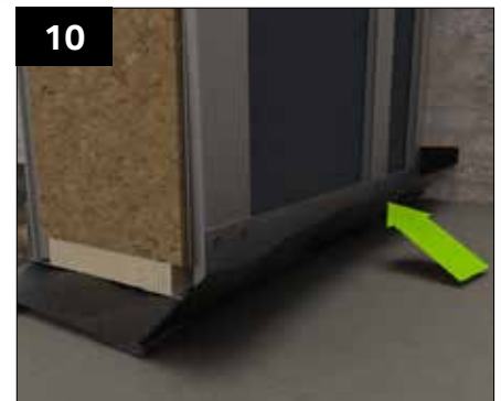
Internally fold up the excess DPC and temporarily fix in place, this can be done with tape or other method.
