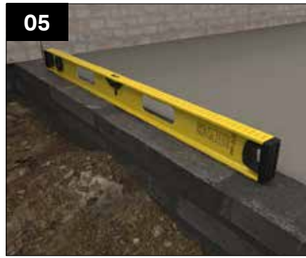
05 Ensure base is level. If required level off with metal or slate shims or a bed of mortar.
